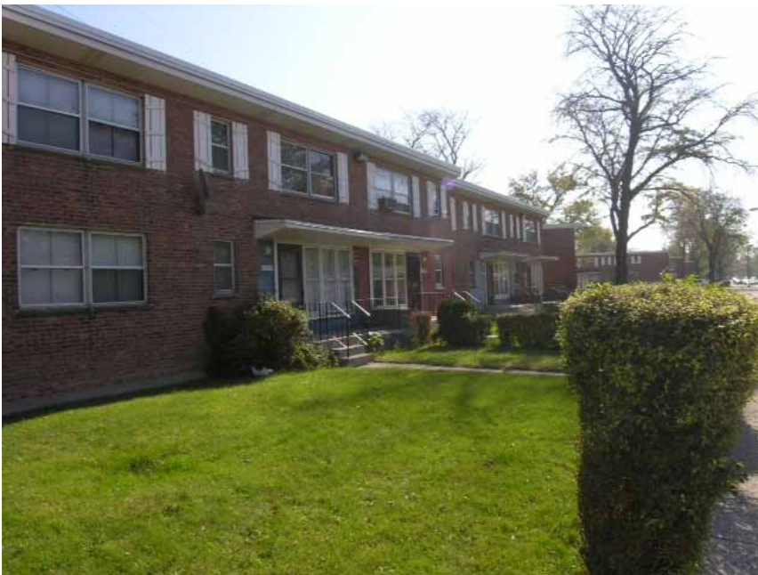
Racine Courts, built in 1950 and converted to co-op in 1968, has stood the test of time.
